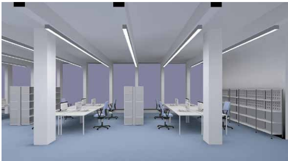
Open-plan office with 8 x 6 LED luminaires
